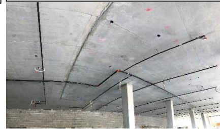
Fire Protection Rough-In
