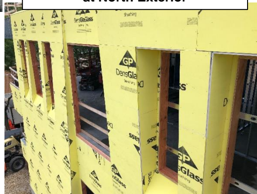
DensGlass & Window Blocking at North Exterior
