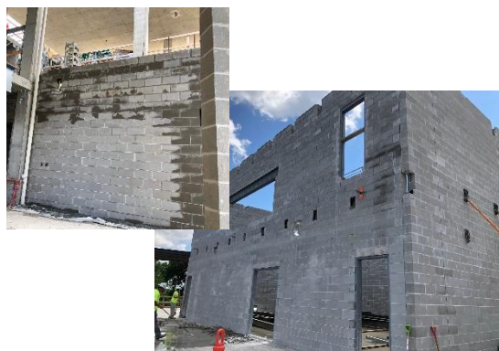
CMU Wall Progress at Black Box & Stair B
