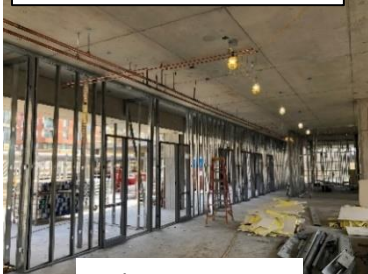
3 rd floor offices
