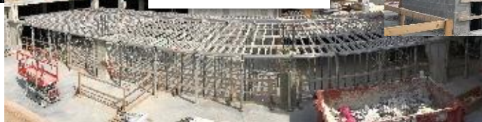
Shoring for L4P4
