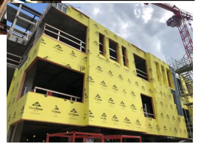
DensGlass at North Exterior
