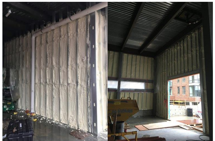
Framing and Spray Foam at the 4 th Floor
