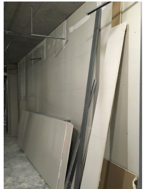
Drywall on 1st Floor
