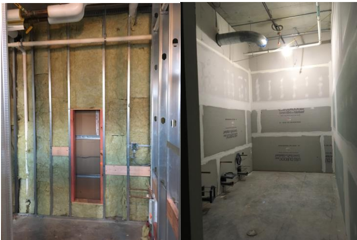
Bathrooms in Progress
